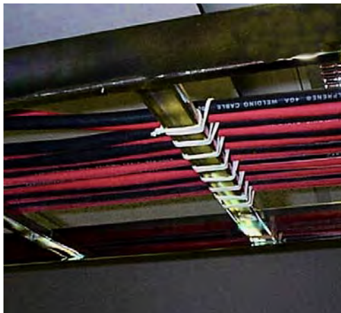
FIGURE 9-17 TELEPHONE COMPANY LACING METHODS
