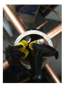
ext, if you are so inclined, use a multimeter to ensure that each leg is electrically separated from the other. Then glue on your top cap. Then proceed to use the outdoor silicone to seal every penetration in the pipe.
